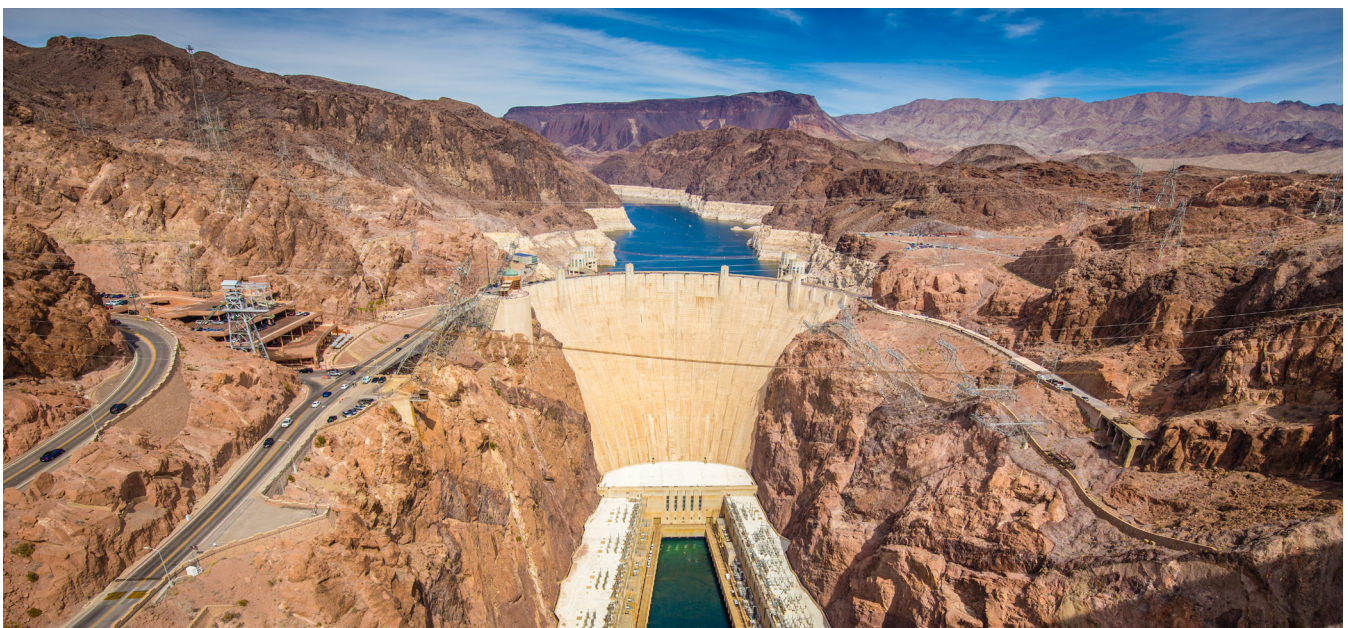
The Hoover dam in the USA provides clean hydropower but negatively impacts the local hydrological system Source: Shutterstock.
