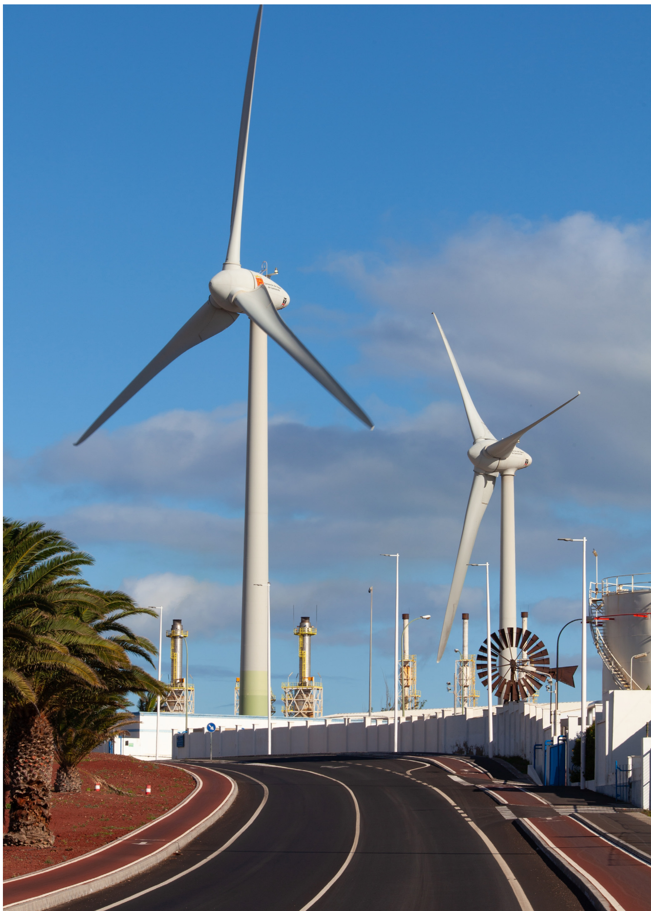
Wind turbines providing electricity for the desalination plant at Costa Teguse, Lanzarote, Spain. Source: Shutterstock.
