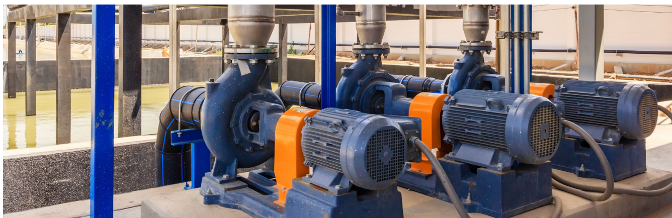
New pumping equipment at an urban wastewater treatment plant can help reduce GHG emissions. Source: Shutterstock.
