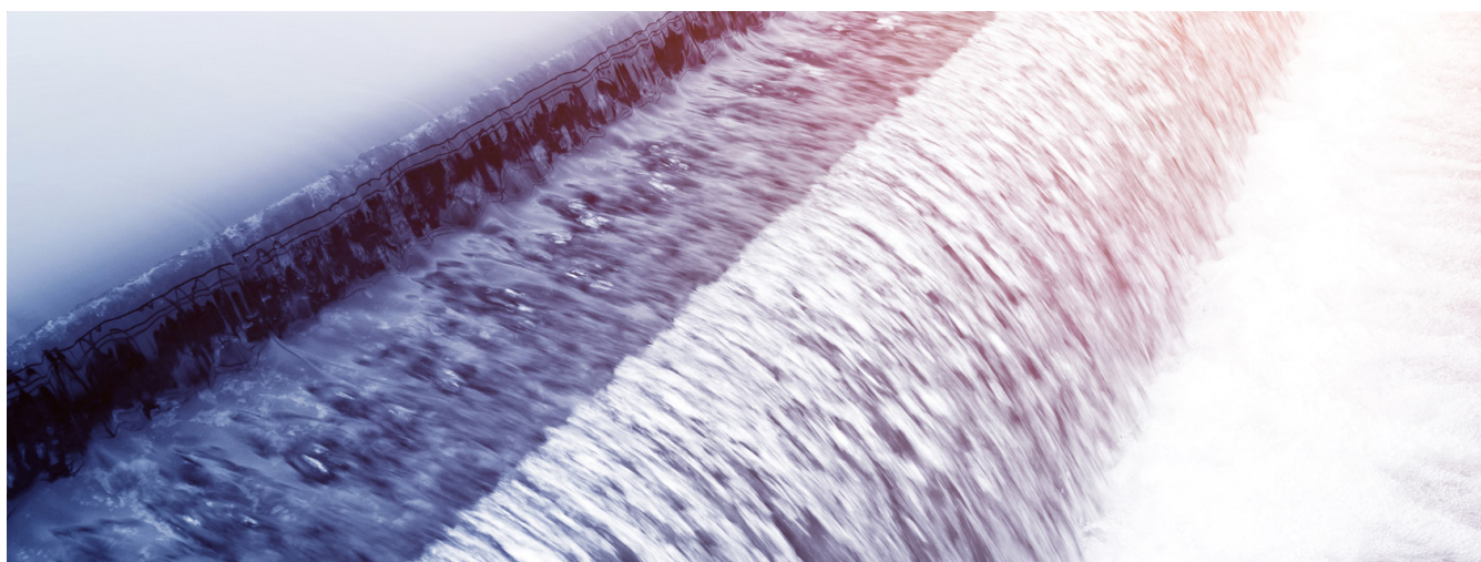
Modern urban wastewater treatment plant. Source: Shutterstock.
