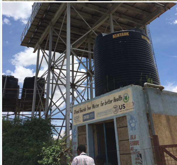
Photo: Water kiosk, including a decentralized treatment facility to remove fluoride, in Naivasha.
