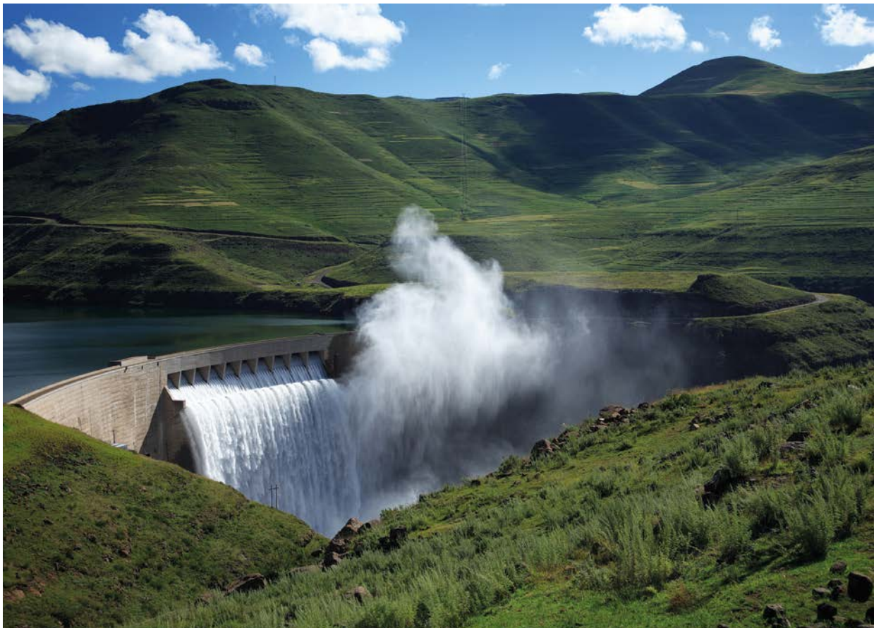
The Katse dam wall in Lesotho, Orange-Senqu river basin. Photo: AdeleD/Shutterstock
