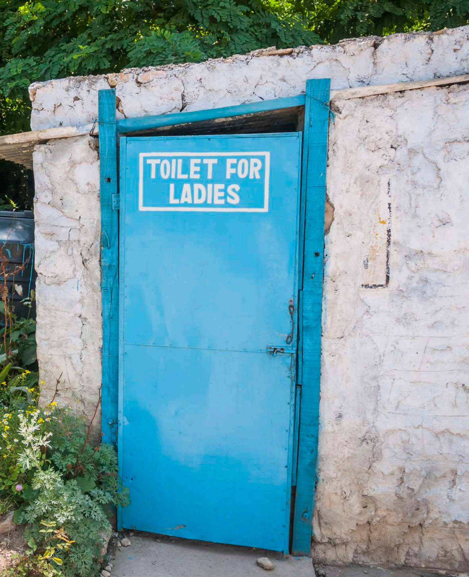
More than 100 million toilets have been built as part of the Clean India Mission. Photo: iStock
